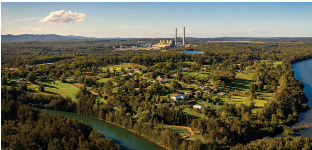
An aerial view of Origin Energy's Eraring power station on the shores of Lake Macquarie, NSW. The plant is now Australia's largest emitter of carbon dioxide, burning 5.2 million tonnes of coal per year from five local mines and releasing nearly 20 million tonnes of greenhouse gases into the atmosphere every year. © Christopher Wright.
