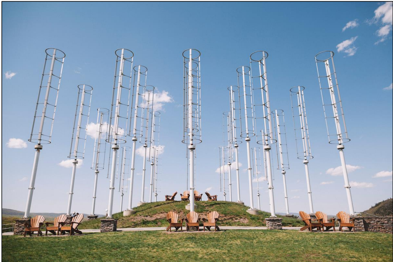
Wind turbines, Quinnipiac University York Hill Campus, Hamden, CT
